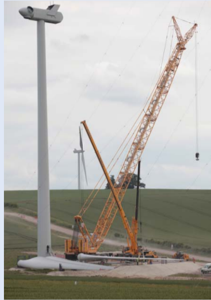
2. The hub and nacelle are put in place.
