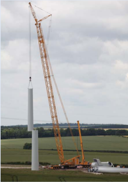
1. The tower sections are connected together.
