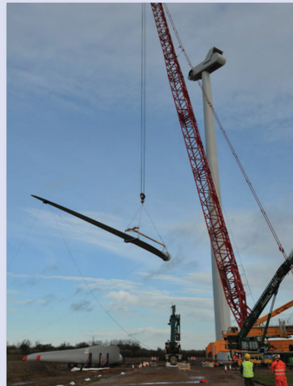
Lifting a turbine blade into place at The Grange Wind Farm, Lincolnshire.
